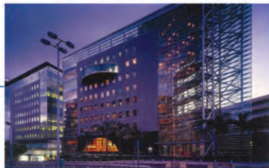
BLOM Bank Central Branch
